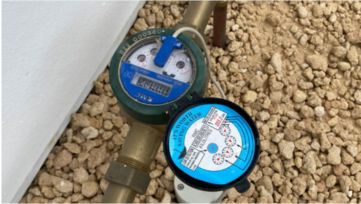
Water meters with electronic monitoring
