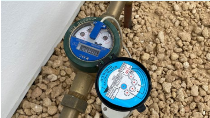
Water meters with electronic monitoring
