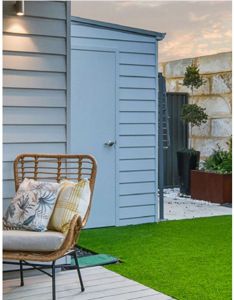
Fibre cement cladded storerooms with GPO and light
