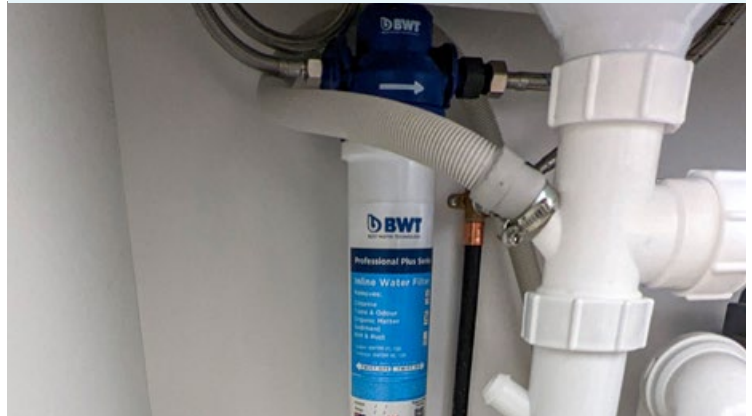
WFA HiFlow inline water filter system
